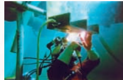
Underwater welding (Photo, courtesy of Hydroweld, Sutton Coldfield, UK)
