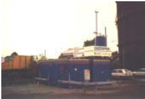
Natural gas compressor for Gothenburg Energi AB.
